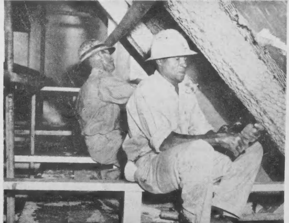
At left, the Cat Plant stack shines after a new coat of aluminum paint. Below at left, William Norris of Process, Thomas Malcolm (then M & C zone supervisor), and Joseph Oduber of Welding discuss a repair job. Below at right, Franciscus de Freitas and Bernard Francis put new insulation on the precipitator.
